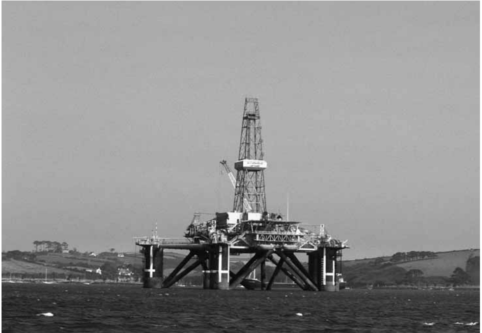
An exploration rig anchored in Carrick Roads in the Fal Estuary, awaiting its next assignment.
